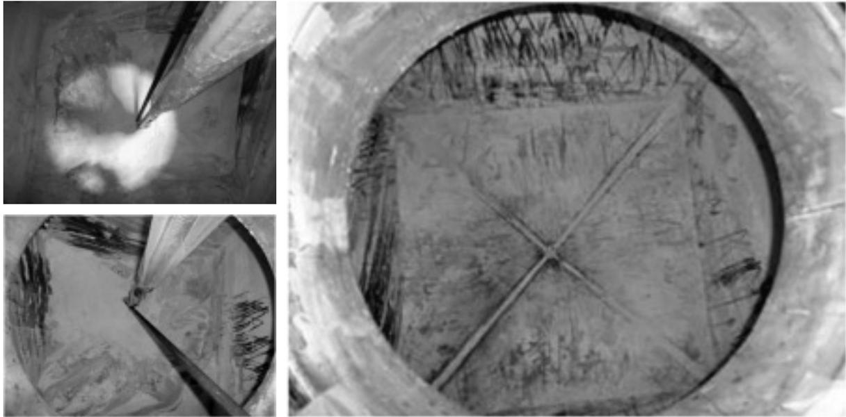
Photo 10 Inside surface of fluidization media storage tanks (Left : during work, Right : after work)
