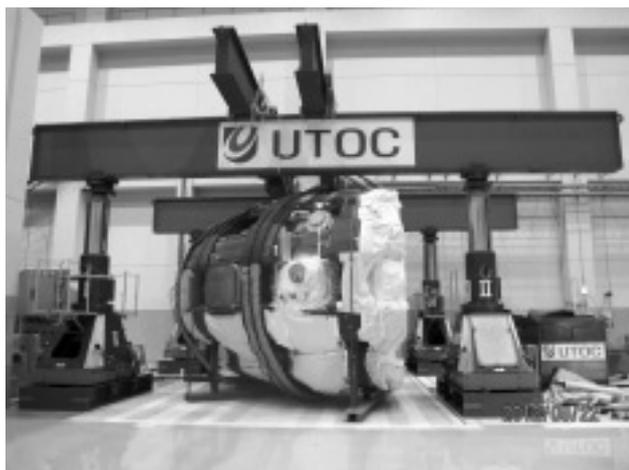
Fig. 17 Setting of vacuum vessel in storage building
