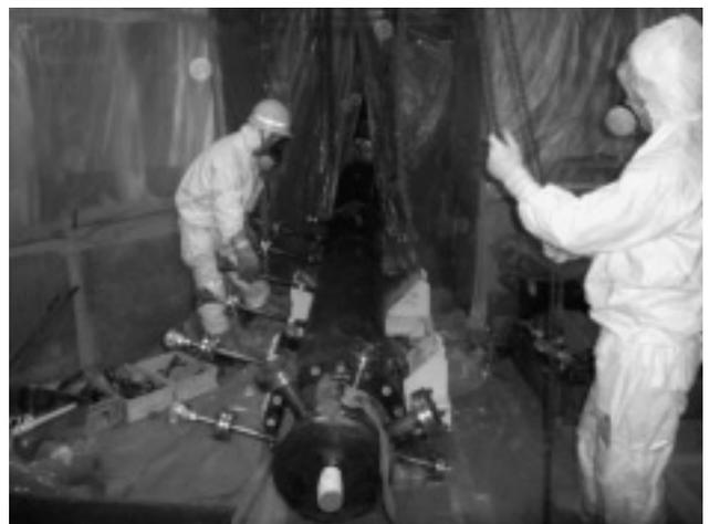
Photo 5 Dismantling work in dewatering conversion room
