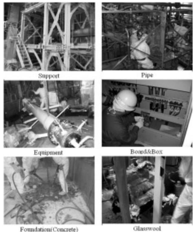
Photo 6 Typical parts of the equipment for dismantling
