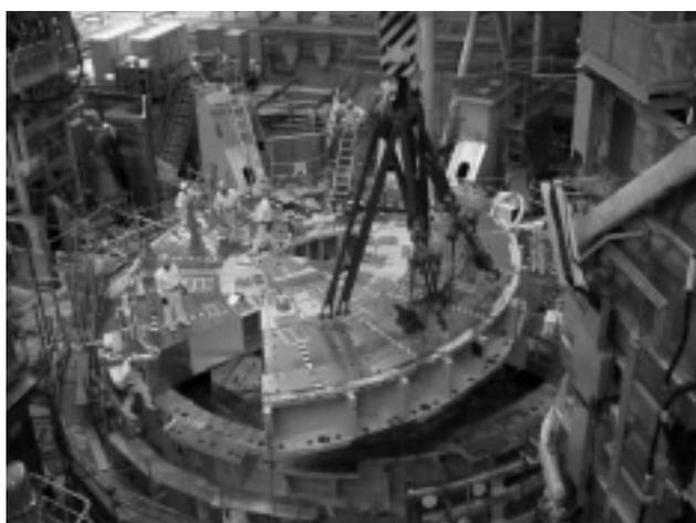
Fig. 18 Disassembly of base frame
