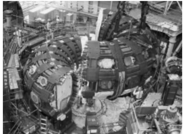
Fig. 15 Lifting of vacuum vessel
