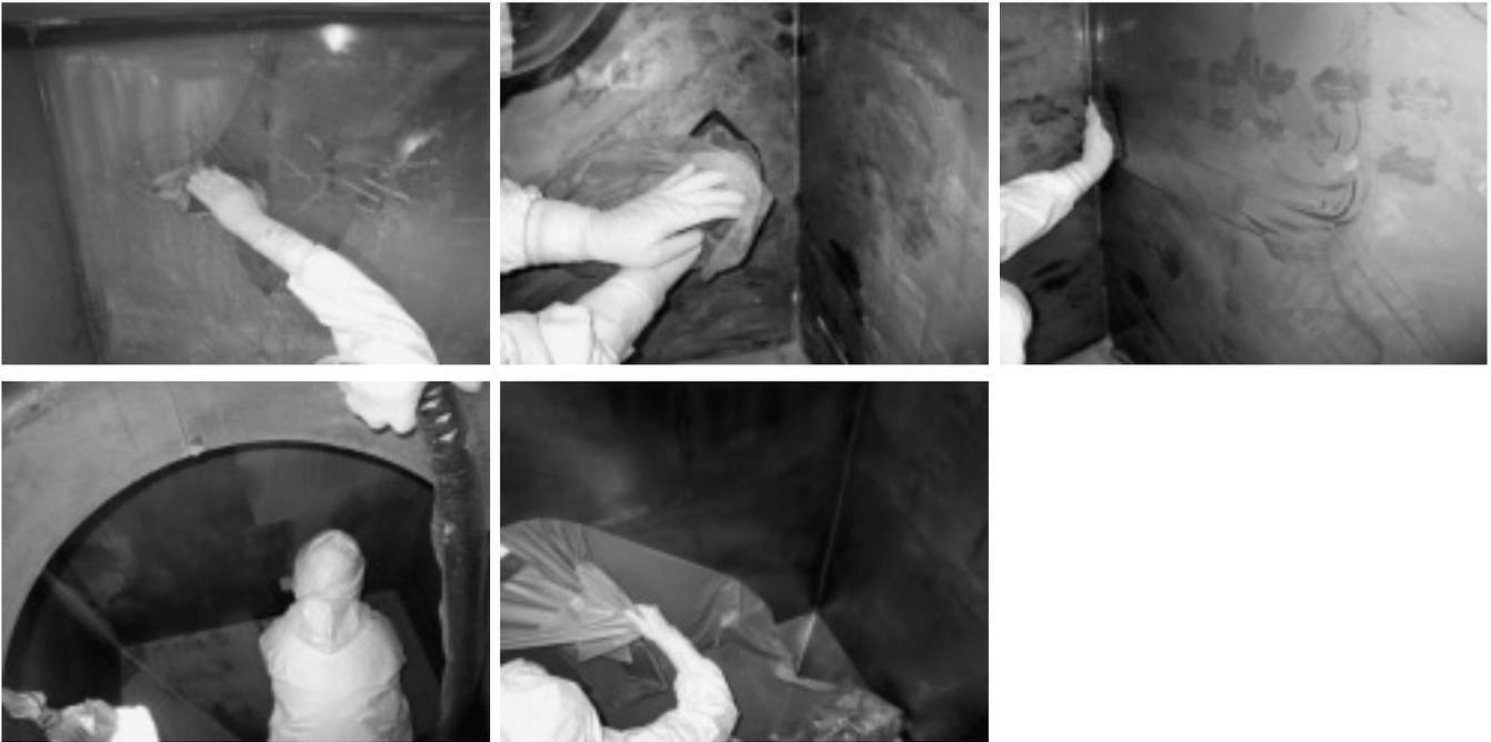
Photo 11 Decontamination process in fluidization media storage tanks
