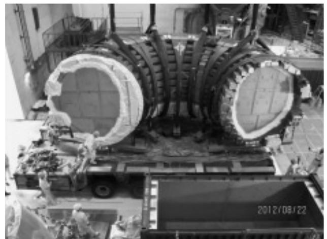
Fig. 16 Transport of half of vacuum vessel
